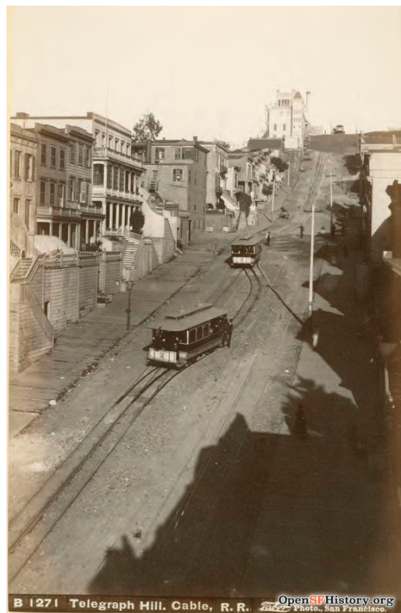
View up Greenwich Street from near Stockton Street. Two Telegraph Hill Railroad funicular cars enter passing track. Layman’s castle at top of hill, circa 1885. (OpenSFHistory/wnp71.0459)
